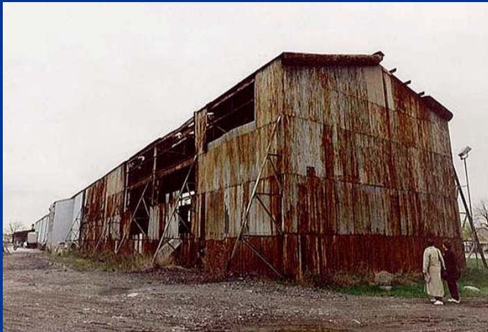
Before - Former Sharon Steel Property, MI
